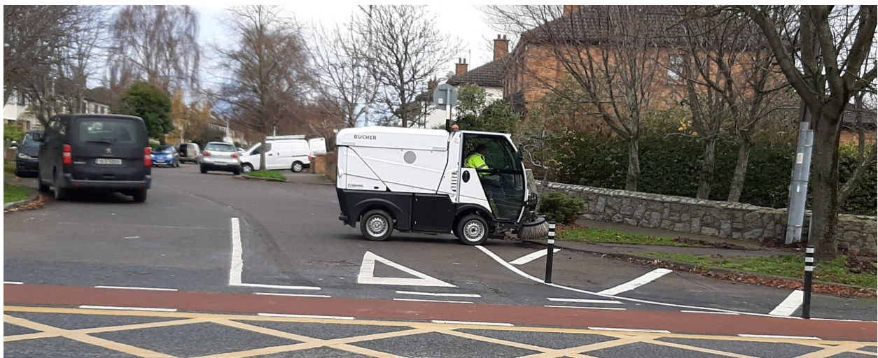
Photo showing wands and line markings used to narrow a side road junction along Goatstown Road, DLRCC. Photo credit: Taney Area Residents' Association
