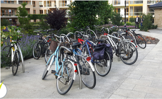
Fig. 24 Bike racks are secure stainless steel, Sheffield Hoop type stands.
