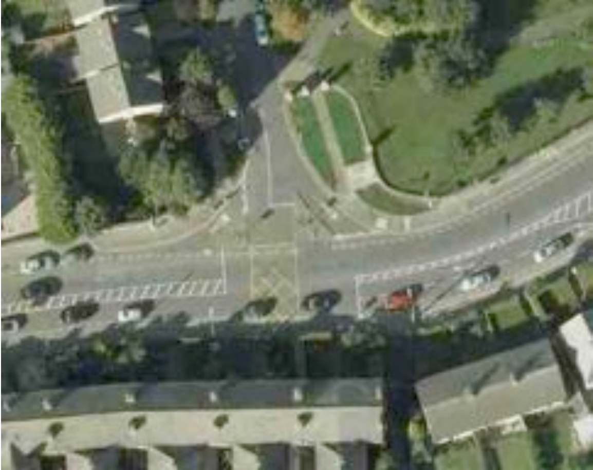
Realign cycle lane. "Yield to Cyclists" sign required
