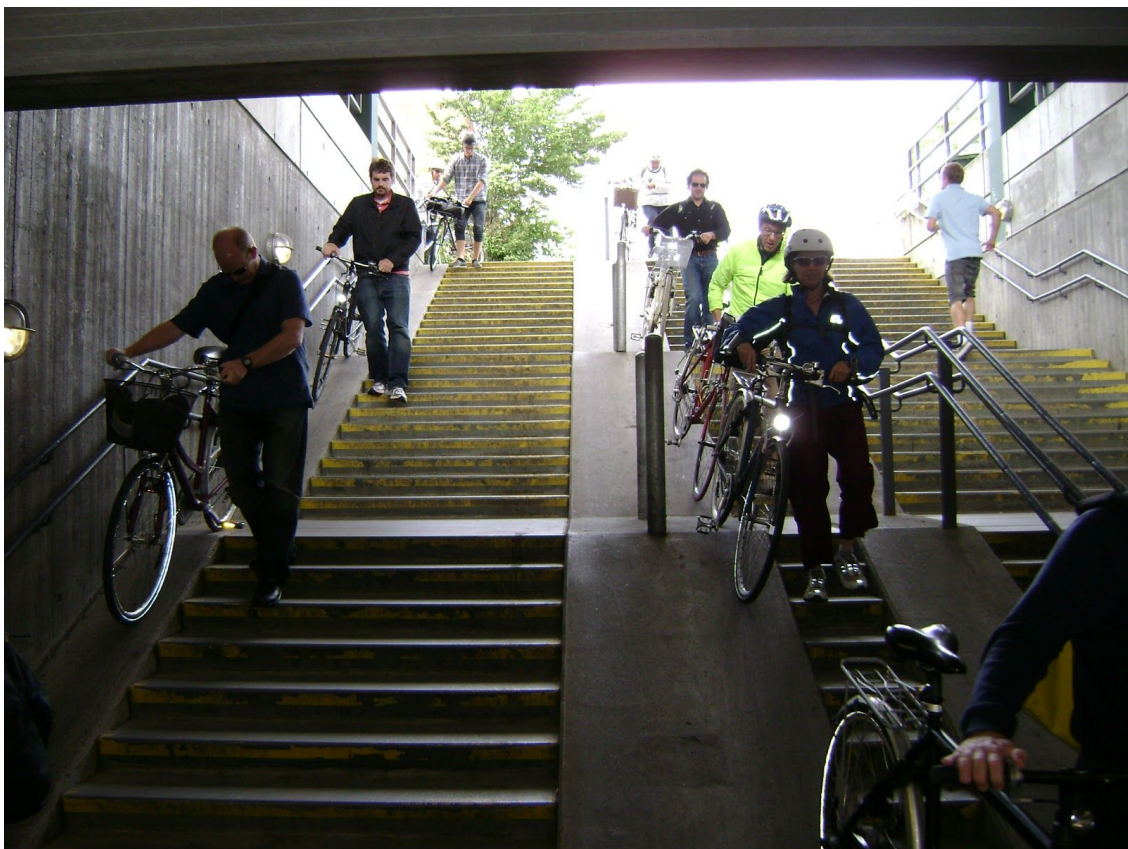
Providing a small ramp on shallow gradient steps can provide cyclists easy access down into an underground stations or to bike parking within the underground station box
