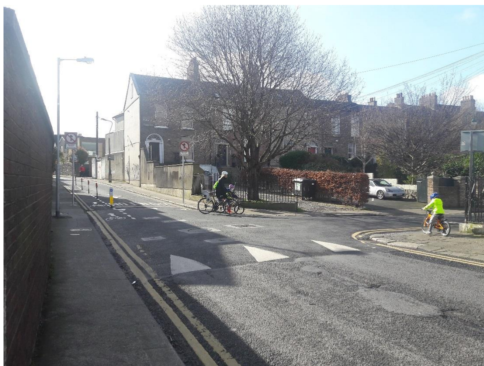
Traffic Calming Measures at junction of Richmond Hill / Mountpleasant Avenue Upper
