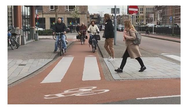
In this design, cyclists and pedestrians cross together, and motor traffic waits / yields for both during crossing phases. At future dates, should the signalised crossings be safe to remove and replace with zebras, this design creates space for "shark teeth" holding zones where turning motorists have full line of sight of crossing pedestrians cyclists with no blind spots to worry about
