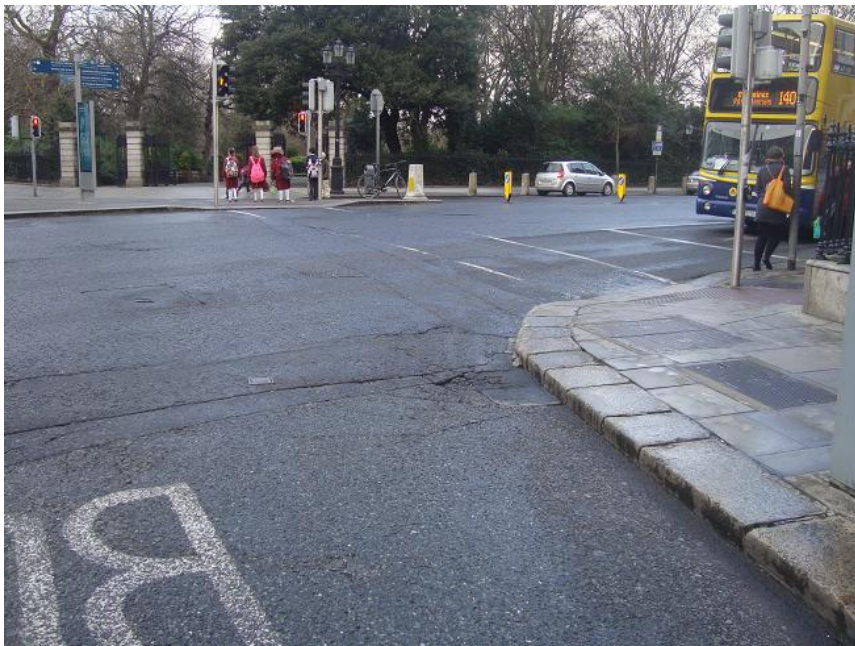
Photo 8 – Poor road surface, ill-fitting manholes and damage to kerbs at St. Stephen's Green East-Leeson Street.
