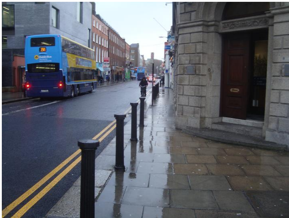
Photo 9 – Substandard width of footpath on Merrion Row.
