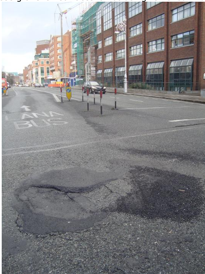
Photo 6 – Severe pothole and debris field at the junction of Earlsfort Terrace at Hatch Street
