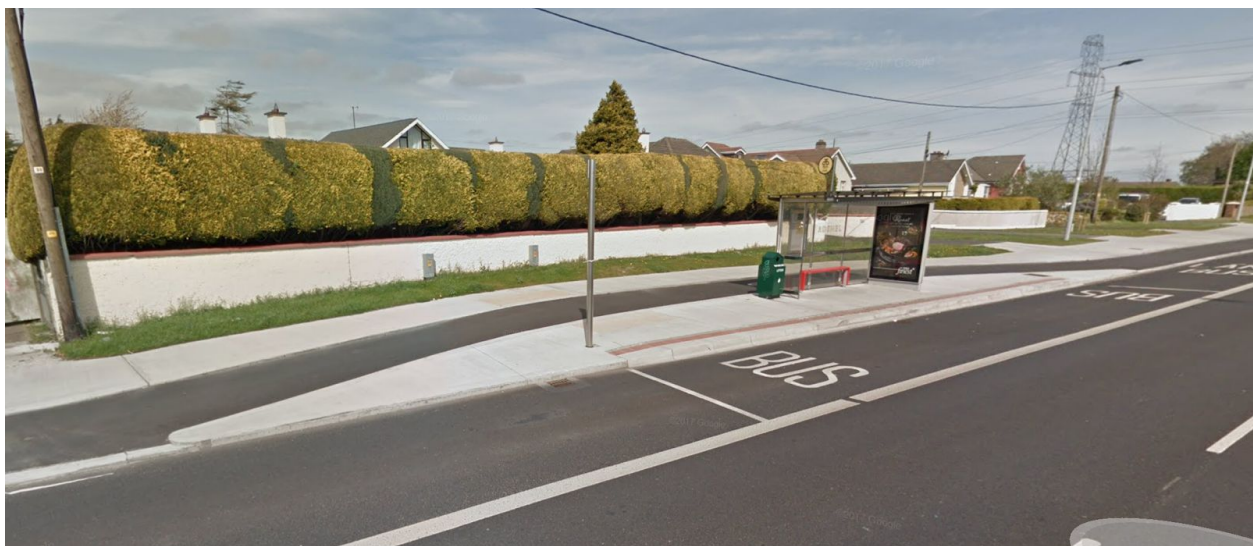
Example of a bus stop with a cycle bypass in Tallaght
